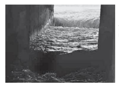
Figure 17. The inside view of the channel. Notice the difference in height between the river bed and the bottom of the bridge (photograph by Shah Karami, 2006).
