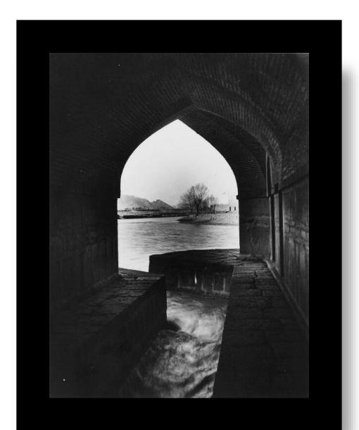
Figure 19. The sluice gate under the bridge. The sluice gate is located under octagonal pavilion called "BygIrbygy" (photograph by Robert Byron [1905-1941], 1933-1934). Fourthly, at the exit of water, the special design of the channels calms the water wave upstream of the Zayandeh Rud River and changes the waves of the water downstream of the river (Shah Karami, 2006).\_(please refer to Figure 20).
